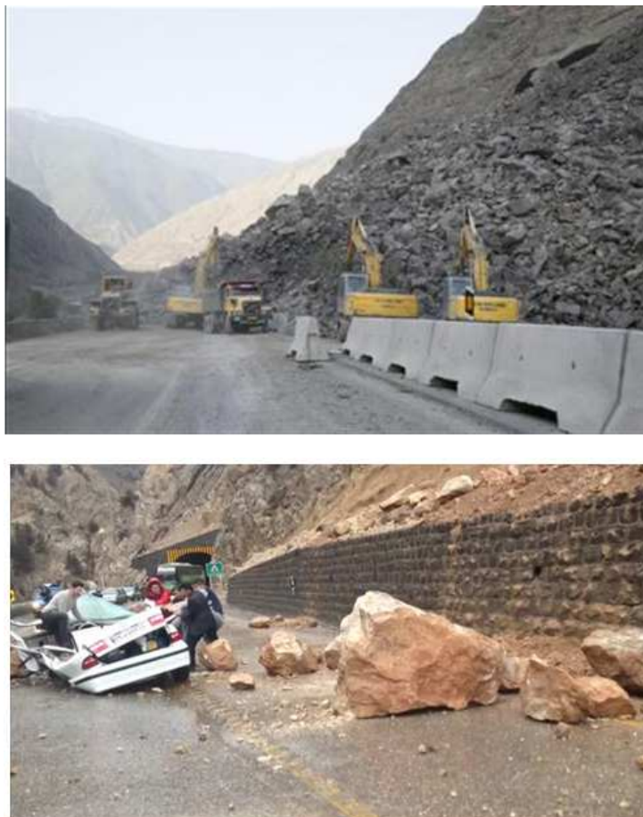
Fig. 3. Rockfall damages in Takavar and Ebtahaj tunnels in 2013
