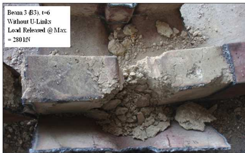
Fig. 7. Crushed concrete in the concrete filled tube beam without any special confinement system at failure
